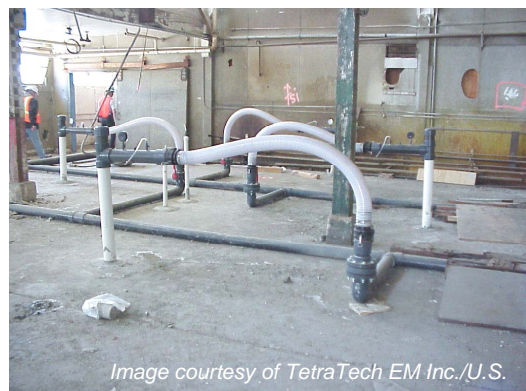
View of pipes for soil vapor extraction (SVE) study at Hunters Point Shipyard, San Francisco, California.
