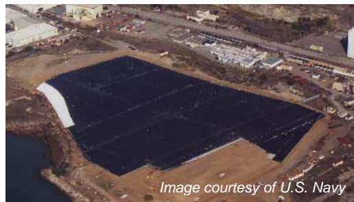
Aerial photograph of landfill cap being installed at Hunters Point Shipyard Parcel E. San Francisco. California.
